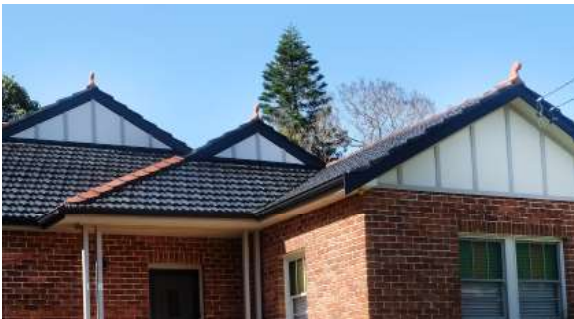
The face brick, roof tiles and light-coloured trims/ eaves of this recent development suit the materials used in the area
