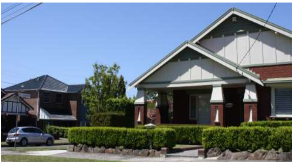
A key characteristic of the area is prominent light-coloured gables that face the street
