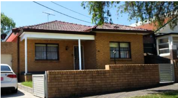
This single storey Inter-War house displays a low pitched roof, brown brickwork and terracotta tiles
