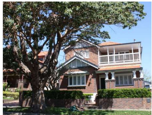
This second storey addition steps back and applies similar materials, proportions and roof forms of the original building
