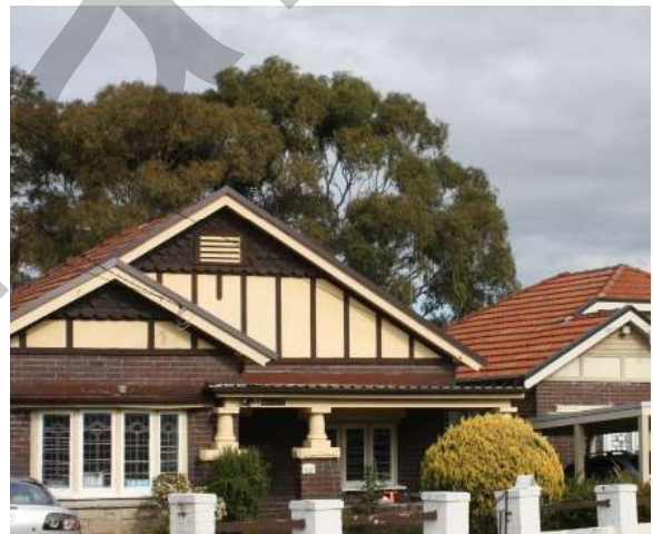
Most buildings in the area have tiled roofs in natural dark red and red-brown colours
