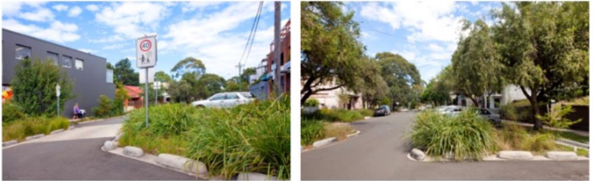
Figure 5-3 Kerbing to allow irrigation of street trees
