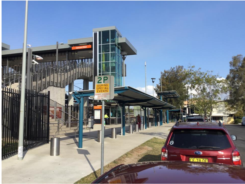
Photo 1: Concord West Station – With existing bicycle facilities in background
