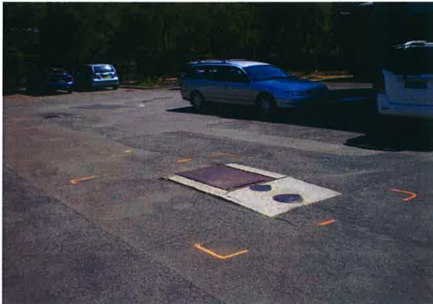
Photo 1: Fill & dip points of underground storage tank at 7 Concord Avenue (painted lines on ground surface indicate approximate extremities of the tank)
