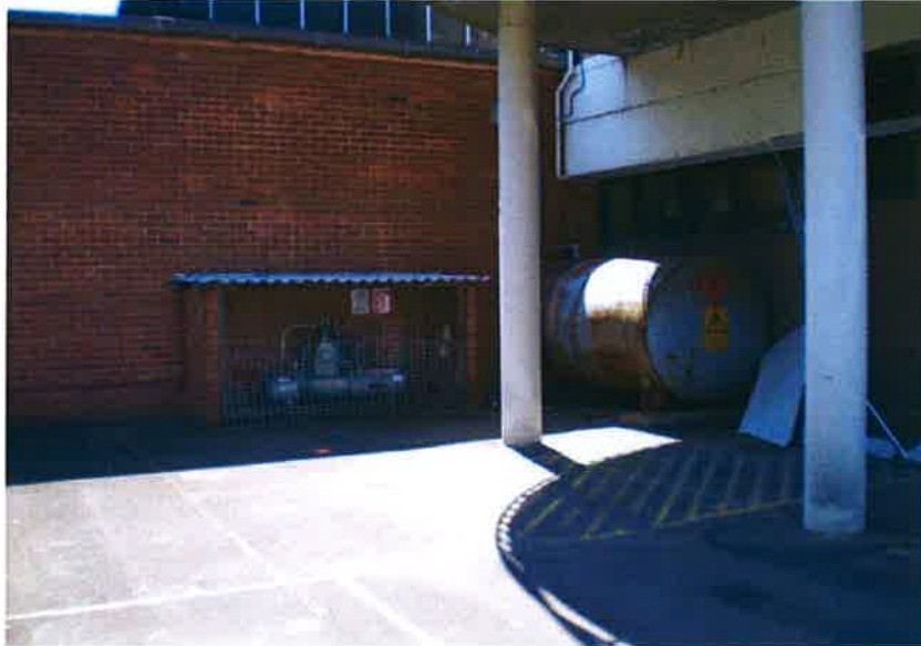
Photo 3: Above ground storage tank for heating oil at 7 Concord Avenue
