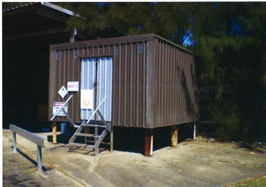
Photo 6: Roofed store at 202-210 George Street
