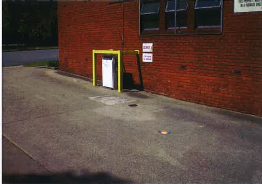
Photo 5: Bowser and fill point for underground storage tank at 202-210 George Street
