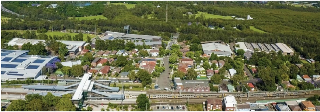
Figure 1: Aerial view of the subject site.
