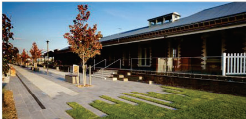
Station forecourt and plaza on Queen street to be upgraded and expanded
