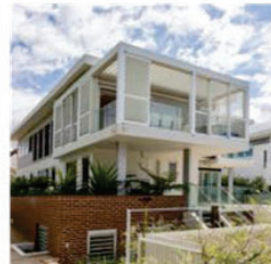
Two storey multi residential building that complements the stand alone nature of neighbouring development.
