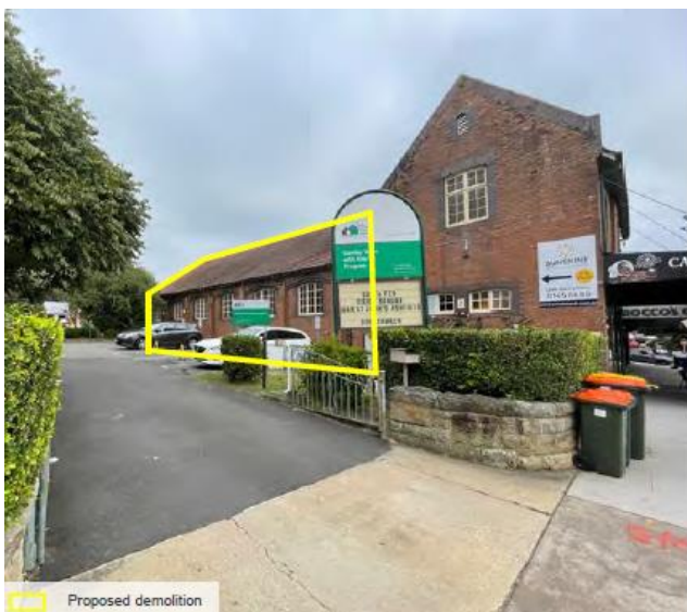
Figure 21: View of St Alban's Anglican Church Hall from Great North Road
