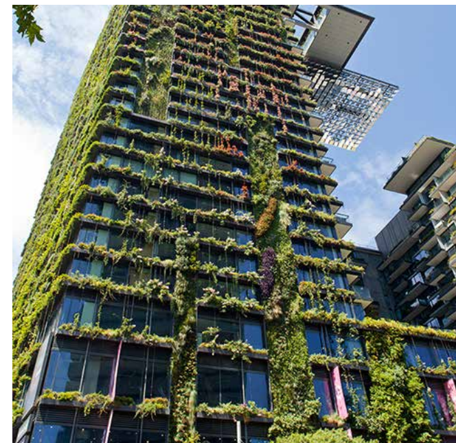
One Central Park's green facade. (Image source: Tensile)
